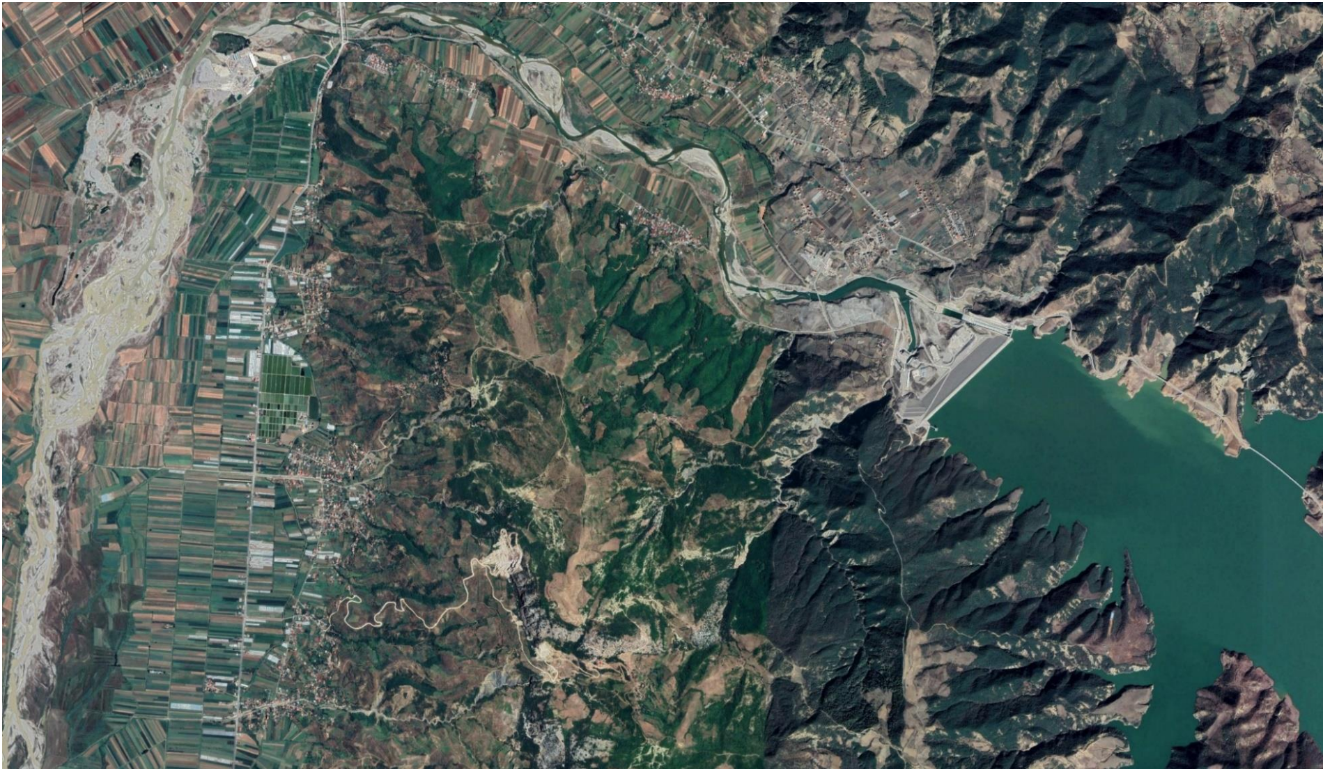
Figure 23: The Devoll river in Albania exemplifies a worst-case scenario: hydropower dam development on a previously free-flowing river with intact hydrological regime and sediment continuum. Now the large impoundment degrades the river from the braided section downstream start (compare also Hauer 2019). The HYMO assessment drop not only for the impounded reach considerably, but also downstream (source: Google Earth, Digital Globe 2019).
